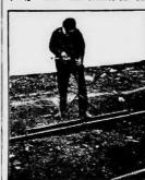
ries renewable saw blade contacts which will not fail to make good contact. The bar may be folded for easy transportation. In operation, a section of the bar is made to span the joint. The central button of the instrument is then rotated until the galvanometer needle at the top comes to 0. The rotated needle then indicates directly on the scale the length in feet of an unbroken rail having the same resistance as the bonded secsame resistance as the bonded section.—From the Scientific American.
