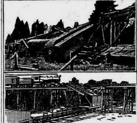
The Passenger Train Broke Through the Sagged Portion of the Trestle and Crashed on to the Work Care Below.
