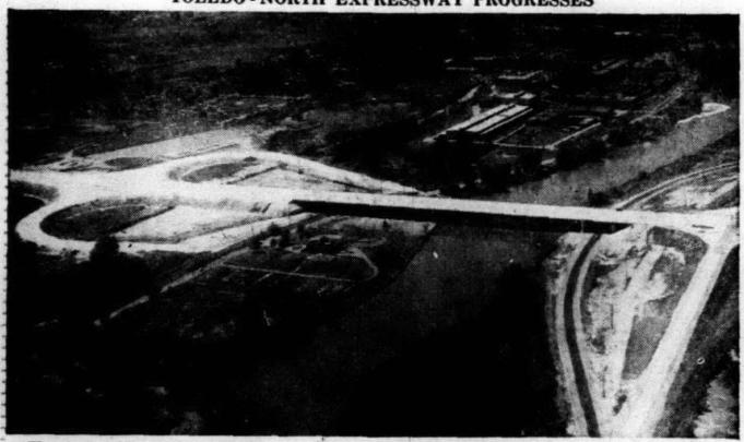
The above bridge recently completed across the Raisin River in Monroe will carry traffic through the east section of the city on the Toledo - North free expressway. This bridge is one of 34 bridges and grade separation structures on this limited access route which stretches for 24 miles. This four-lane divided highway is being built at a cost of some \$27,000,000 in federal, state and City of
