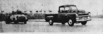
Here's the scientific way to measure the actual pulling power a truck can deliver to its rear wheels. All three low-priced trucks were hooked up, one by one, to a special dynamometer truck. Each was comparably equipped and test-loaded.
