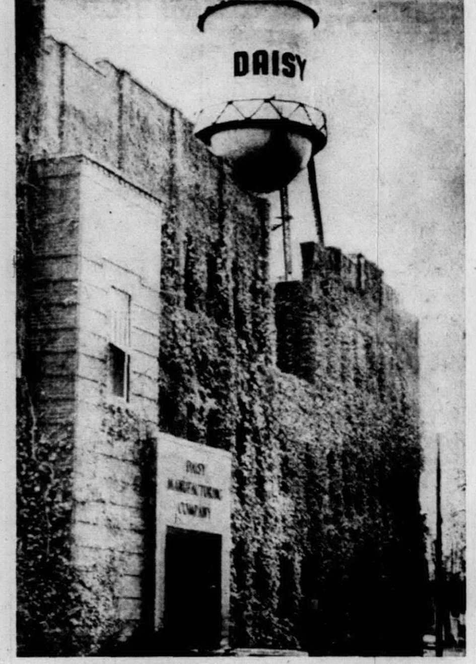
UNION STREET has been the home of Daisy Manufacturing since its early days. The brick, vine-covered building has undergone many alterations and has had numerous additions through the years. Today 600 people work there. Daisy hopes to sell the building.
