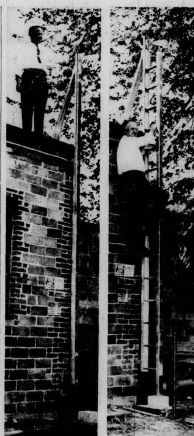
INVENTOR Dan Spence demonstrates his first fire ladder installation at Saxton's Farm Supply. Standing on the roof, he pulls a handle (left) on top of an object that looks something like a down-spout. In an instant a ladder springs forth and the inventor climbs down. The ladder has been given city approval. Offices are located on the second floor of the building's front
