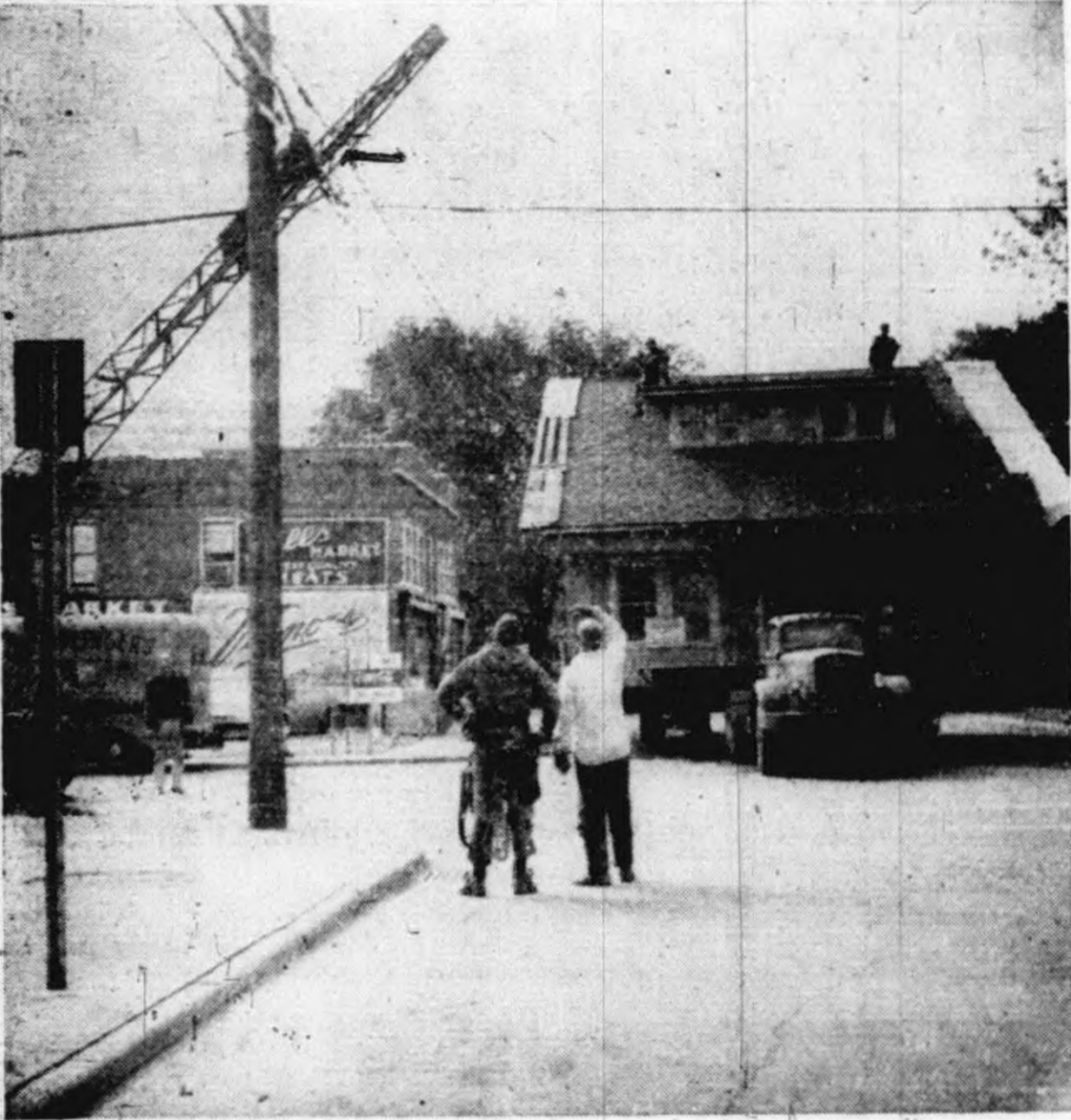
GANGWAY. a house is coming down the street. This one moved from N. Main St. near Mill, down Starkweather Ave. and to a new resting place at the north end of Mill. Here, as it passed Mill's Coffee Shop, workers atop the roof were handed coffee for their coffee break but the house kept on rolling. Utility workers preceded the house with a rig to raise all the low wires. A new Beyer Drug Store is being built on the site where this house and another stood.
