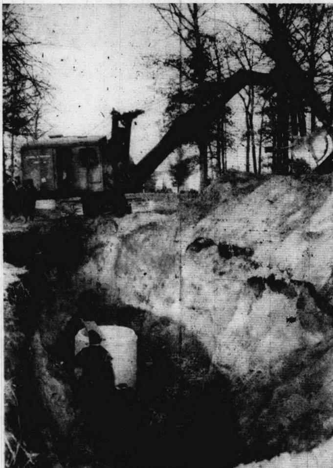
THE MIDDLE of Gold Arbor Rd. nowadays looks like it has been bombed out but this is the type of work that has been going on in Plymouth Township since March. Workmen are shown building up a manhole in the sanitary sewer system that is expected to be ready in several more months.
