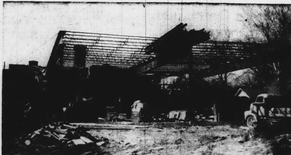
**GOING UP** fast these days is the addition being built to the Plymouth Post Office. The I-beams weighing seven and a half tons each were put up last week and brick work is now progressing. The addition will double the work space of the building. It will be completed this summer.
