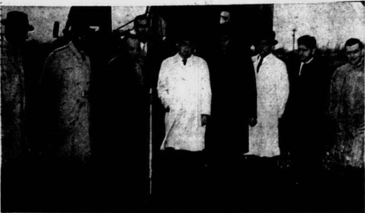
GROUND-BREAKERS —Garden City officials and executives of General Motors' Chevrolet Division joined Gene Merollis Friday in a ground-breaking ceremony for a new sales and service headquarters on Ford road, near Merriman. Present, were (left to right) Russell Sessions, Chevrolet district manager; T. J. Rademacher, zone sales and promo-
