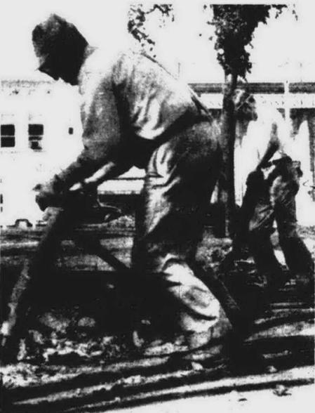
**WORKMEN WERE** hard at it last week breaking up curb in preparation for the installation of sidewalk around the outside edge of Kellogg Park. D.P.W. Superintendent Joseph Bida said plans call for a five-foot strip of sidewalk all the way around the park.
