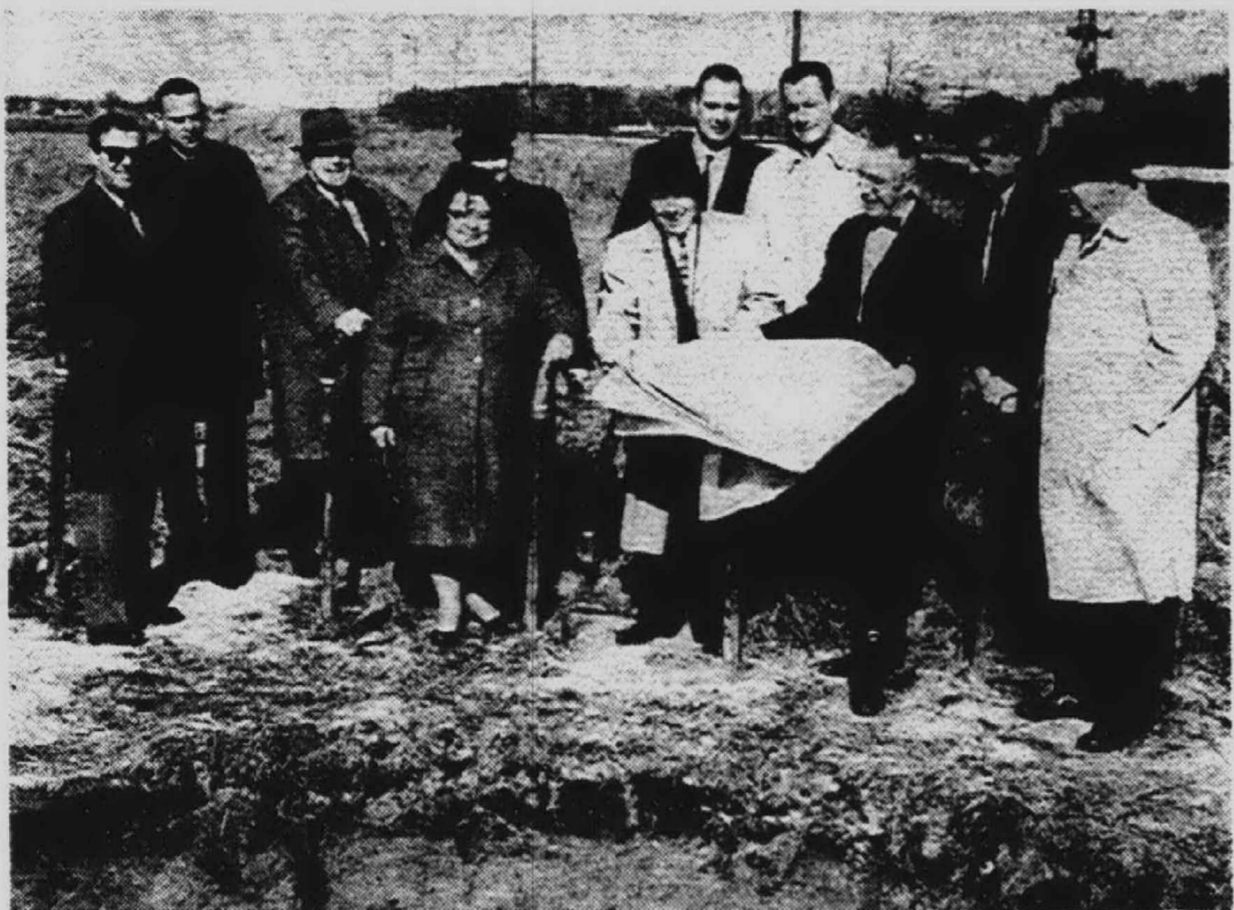
STUDYING PLANS for the Joy Road leg of the $735,000 sewer project in Plymouth Township are officials from the Township, City of Plymouth and the contracting firm. Work started Monday on Joy Road near Haggerty. The group includes: (from left) Contractor Don Gargaro, Robert Rochon from the Gargaro Co., Township Clerk C. Veach Sparks, Township Treas-
