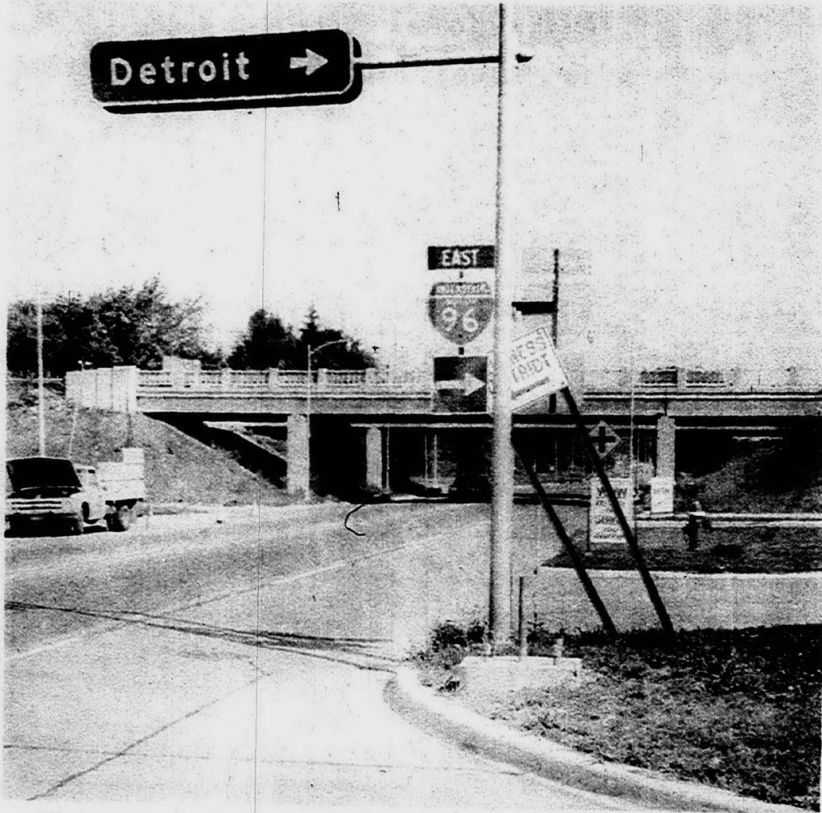
"There are three poles close to the road, and one is in a new two-foot-wide base. A driver going by is within inches of death. They own all this property up to a foot the other side of the sidewalk, so
