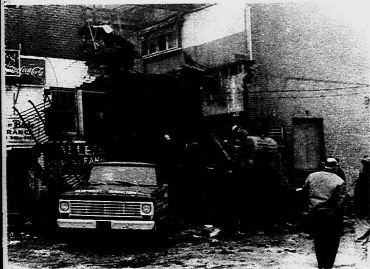
REMOVING TRACES OF FIRE: In the midst of last Monday's fog, the demolition contractors moved in to start work on clearing the debris from the recent Penniman Building fire. Shown in the photo are the men at work and the twisted girders--evidence of the extreme heat.
