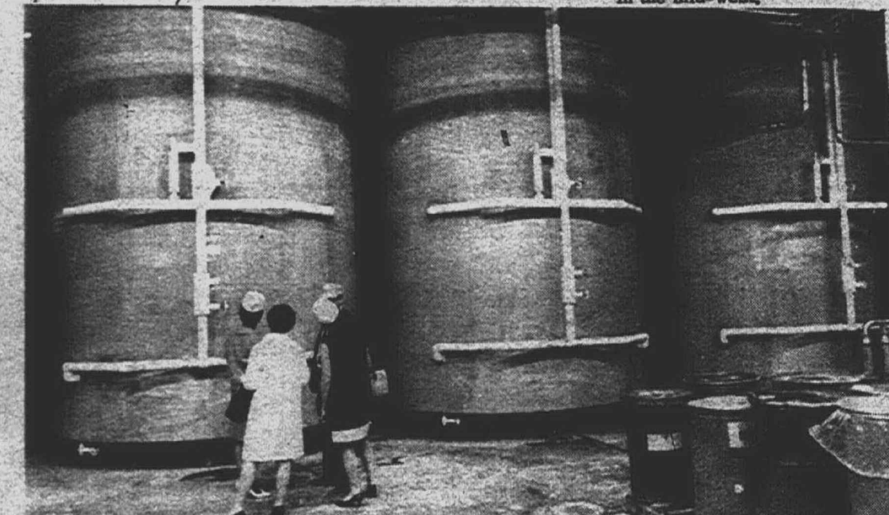
HIGH-RISE STORAGE — Each of these storage tanks goes four stories up and holds 25,000 gallons of milk.
