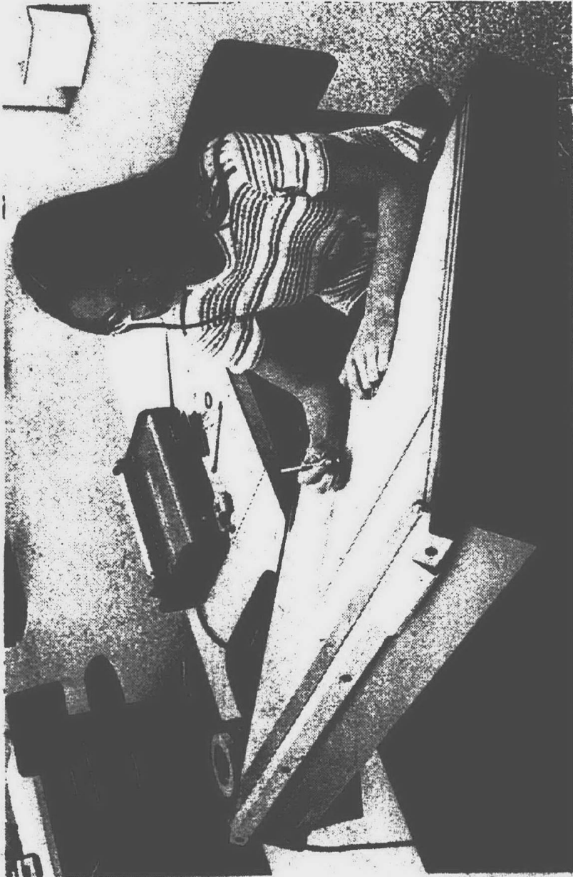
2 Copy is waxed and placed on grid sheets exactly as specified by the advertiser or editor.
