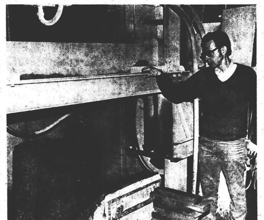
GETTING A FACE LIFTING - Here's an old fashioned tombstone going through the process of rejuvenation. Jim Allenstands by, watching the revolving chain and carborundum cutting off the antique lettering. This is done automatically and the cut averages six inches an hour. (Observer photo by Bob Woodring)
