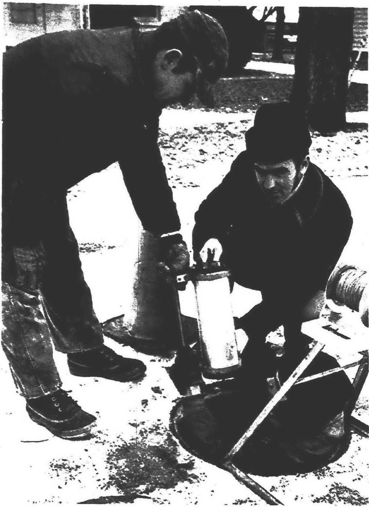
PRIOR TO THE SPRING PAVING of several streets, the sanitary sewers running under them are being photographed to see if any repairs are needed. The 35 mm camera that's doing the job is encased in this metal cylinder. Lowering it into a manhole on Harding for the DPW are (from left) Bob Hastings, Director Kenneth Vogras and Ken Oosterhouse. (Observer photo by Bob Woodring)
