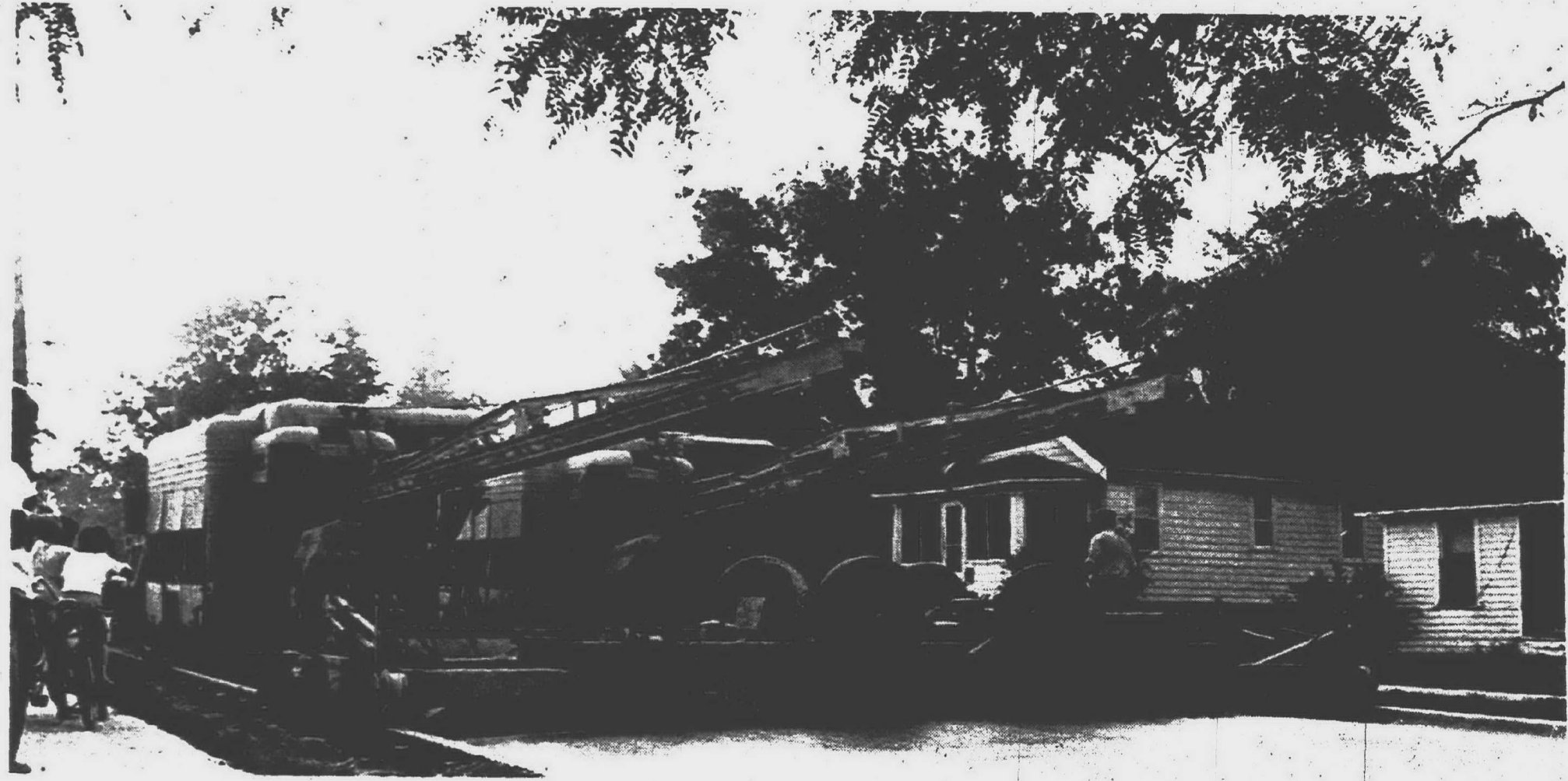
CHANGING THE FACE OF PLYMOUTH -- This giant concrete spreader has been put to heavy use in the past week giving many streets a face lifting in the new paving program.
