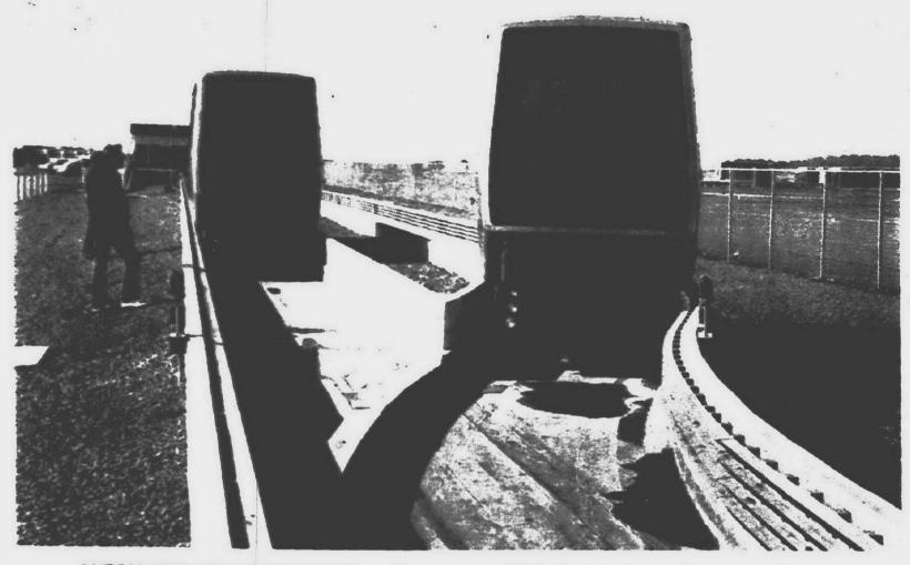
**AUTOMATED TRANSPORTATION — One** of the two vehicles in the Bendix "personal rapid transit" (PRT) system at Transpo '72 at Dulles International Airport switches past the second
