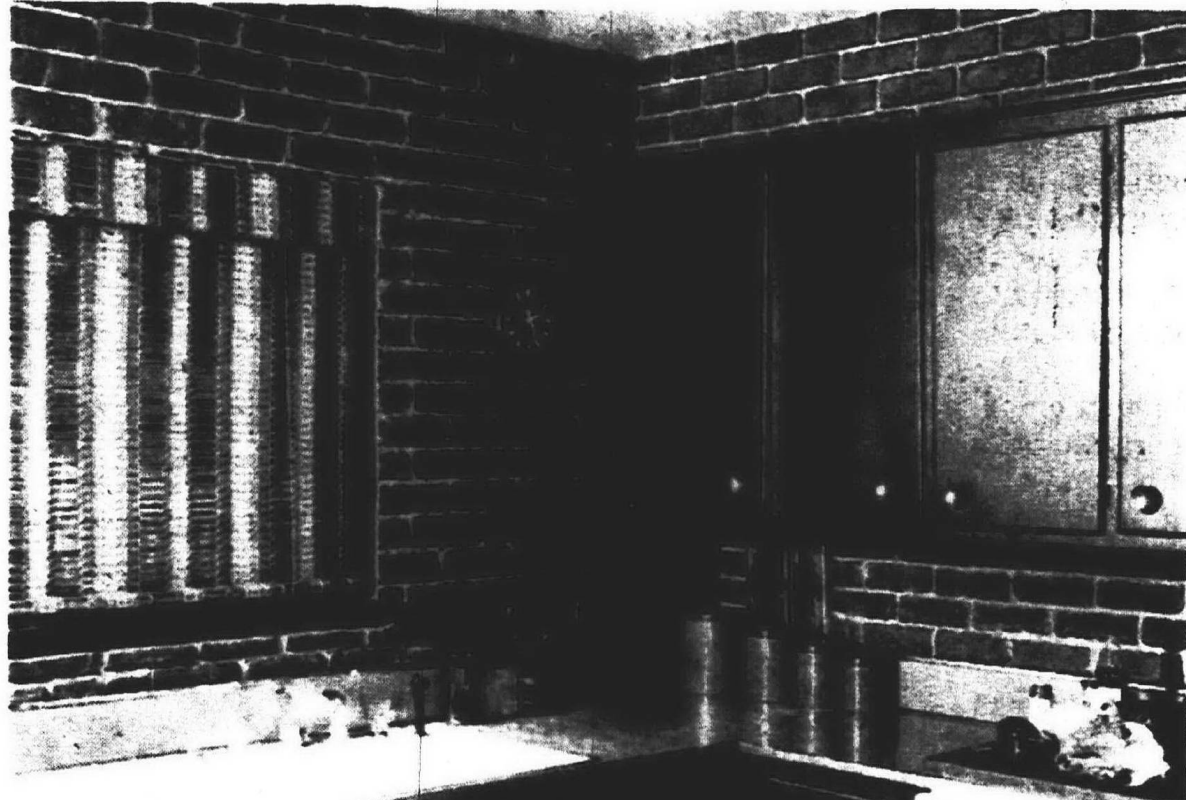
SIMULATED BRICK kitchen is the weekend work of a home handyman using only simple household tools. The "bricks" are made of crushed stone and fiber glass and come in easy-to-install panels.
