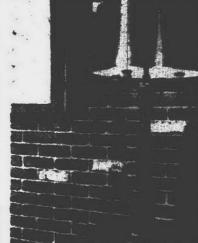
MADE FROM crushed stone and reinforced with fiber glass, panels have the look and feel of brick. Each panel covers about two square feet. Installation is both easy and
