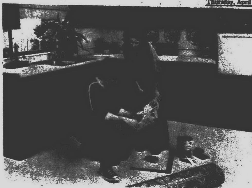
FIRST STEP was careful reading of the instructions. Special equipment included a carpenter's square, chalk line, adhesive, trowel, knife and scissors.
