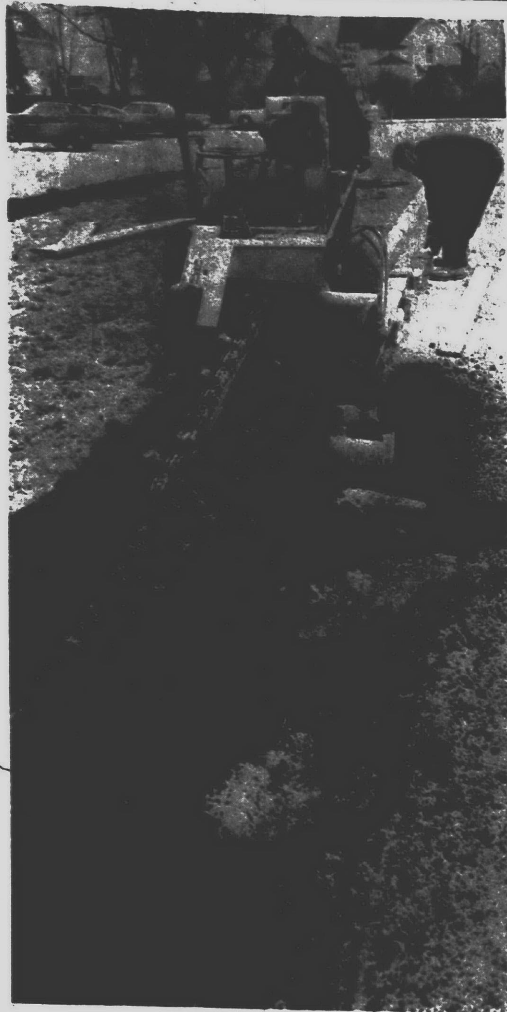
MAN'S GENIUS can conquer any obstacle — just ask the Plymouth DPW workers who were laying sprinkler lines around city hall and ran into a problem. Because the lines were running along the curb of the island on Church Street, the ditching machine couldn't be used. But, someone figured, if you laid down cement blocks with a board over them, the make-shift scaffold would allow the machine to ditch along the curb. (Staff photo by Bob Woodring)
