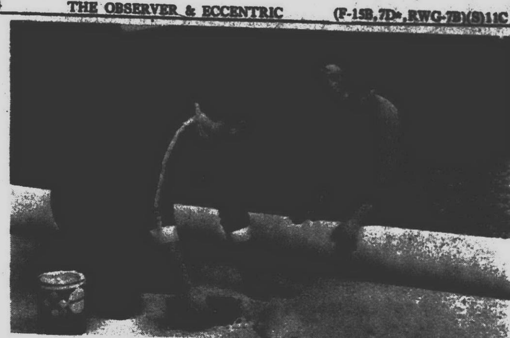
RETURN MATERIAL to room where it is to be installed and put in place. Roll back one half of material, spread adhesive, unroll material onto adhesive while still wet. Repeat same steps with remainder of material to finish job.
