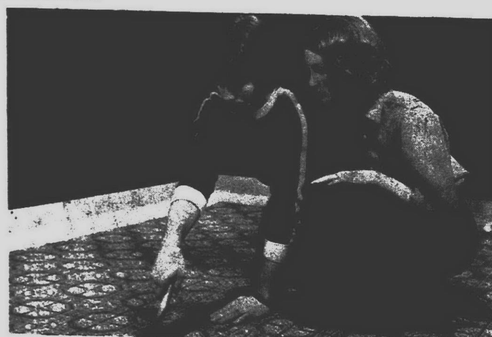
AFTER TRANSFERRING measurements from chart to flooring material, cut along chalk lines using sharp knife and straight edge. Do transferring of measurements and cutting in some room where material can lie flat. Cardboard under cut lines will protect knife blade and surface underneath.
