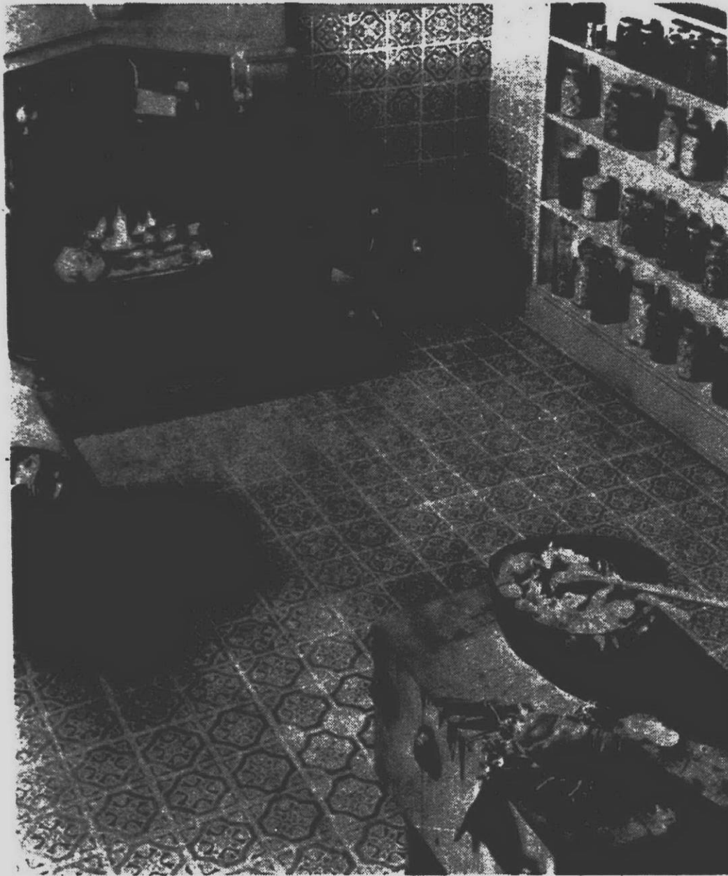
MATCHING wainscot is ideal in kitchens. It will not chip when bumped by furniture; fingerprints are quickly wiped off. The tile wears much better than wallpaper and is easier to apply.
