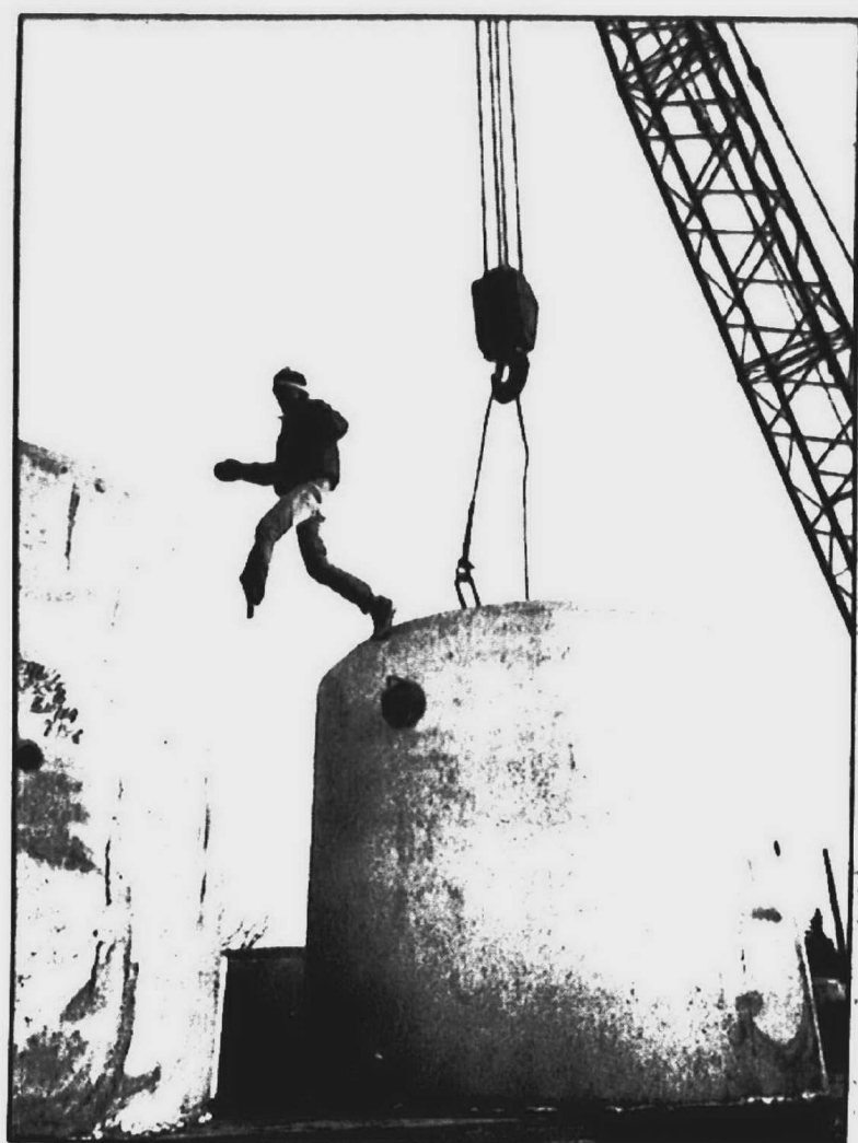
Last week drainage tiles were placed into position. This week crews covered the tiles.
