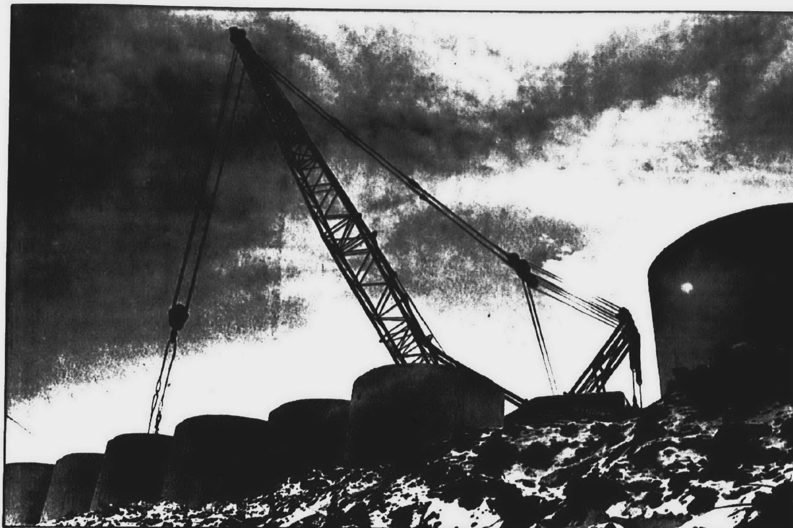
This huge crane is positioned to lift tiles into the Tonquish.
