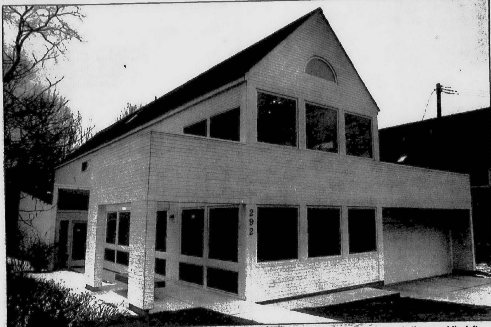
The two-story center section plus everything in the foreground is new, the small section at the back, seen in the rear at the left, is the original house.
