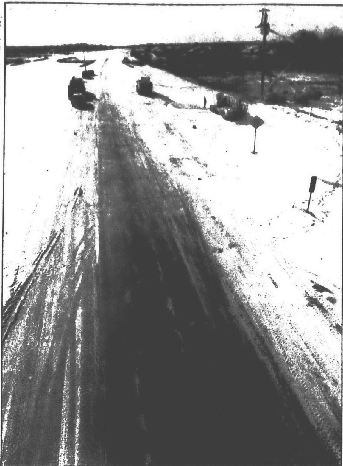
A Detroit Edison crew repaired a power line on the southbound lanes of I-275 in Canton Tuesday while drivers scrambled to find alternate routes.
