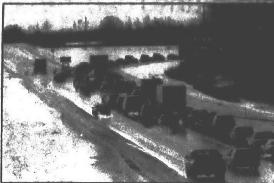
Southbound drivers on I-275 were forced to get off onto Ford Road in Canton Tuesday so Detroit Edison crews could repair a fallen power line.
