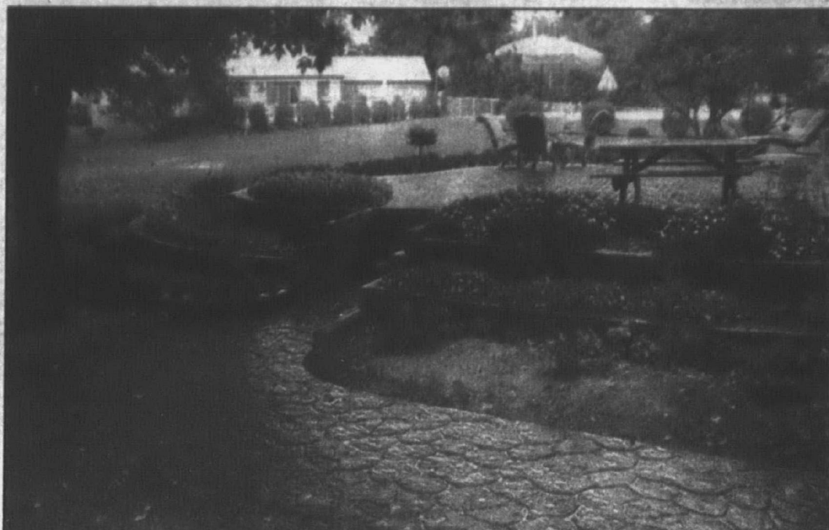
Stamped concrete can offer a less expensive option to paving stones, slate, brick and cobblestone that also gives an attractive alternative to standard pavement.
