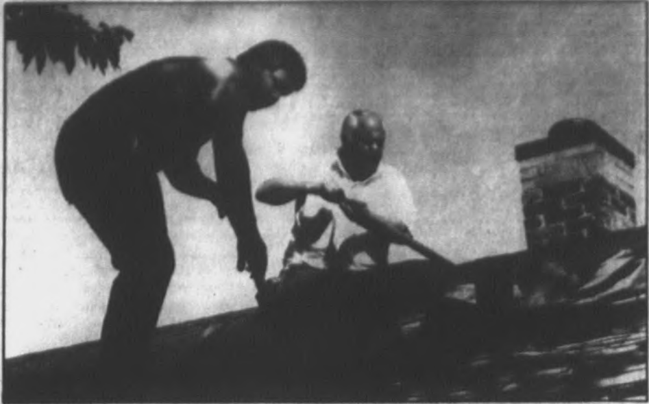
Dan and Carson Coonce rip off the old roofing.
