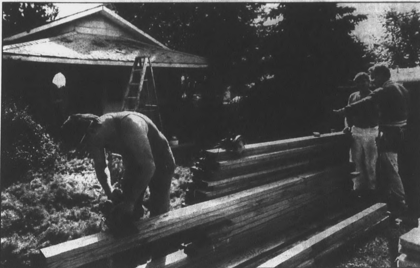
John Meadows cuts a timber for the new porch.
