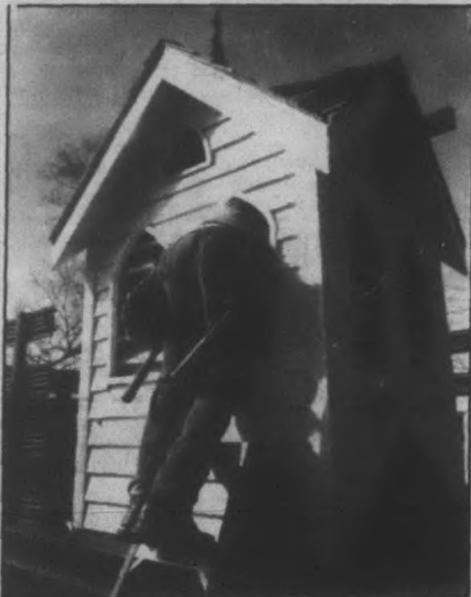
One of the workers checks the interior of the cupola.
