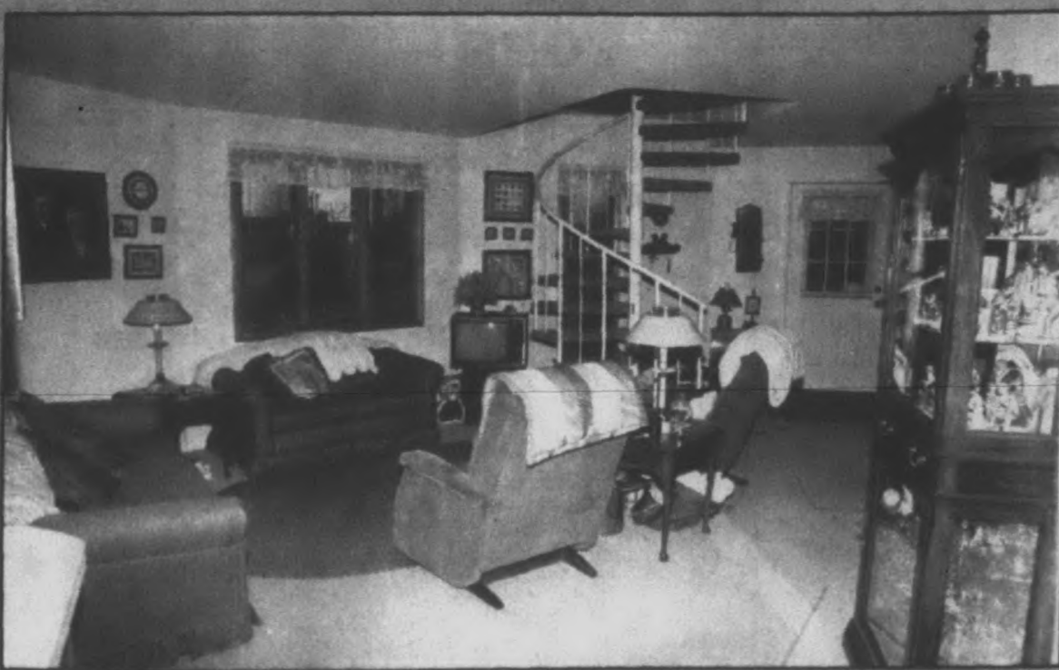
Left: The Eagle's Nest House is made of 14 individual sides, or panels. Each panel is drywalled together to form a cove, giving the interior a round feeling. Elimination of angled walls results in greater air circulation and more useable living space.
