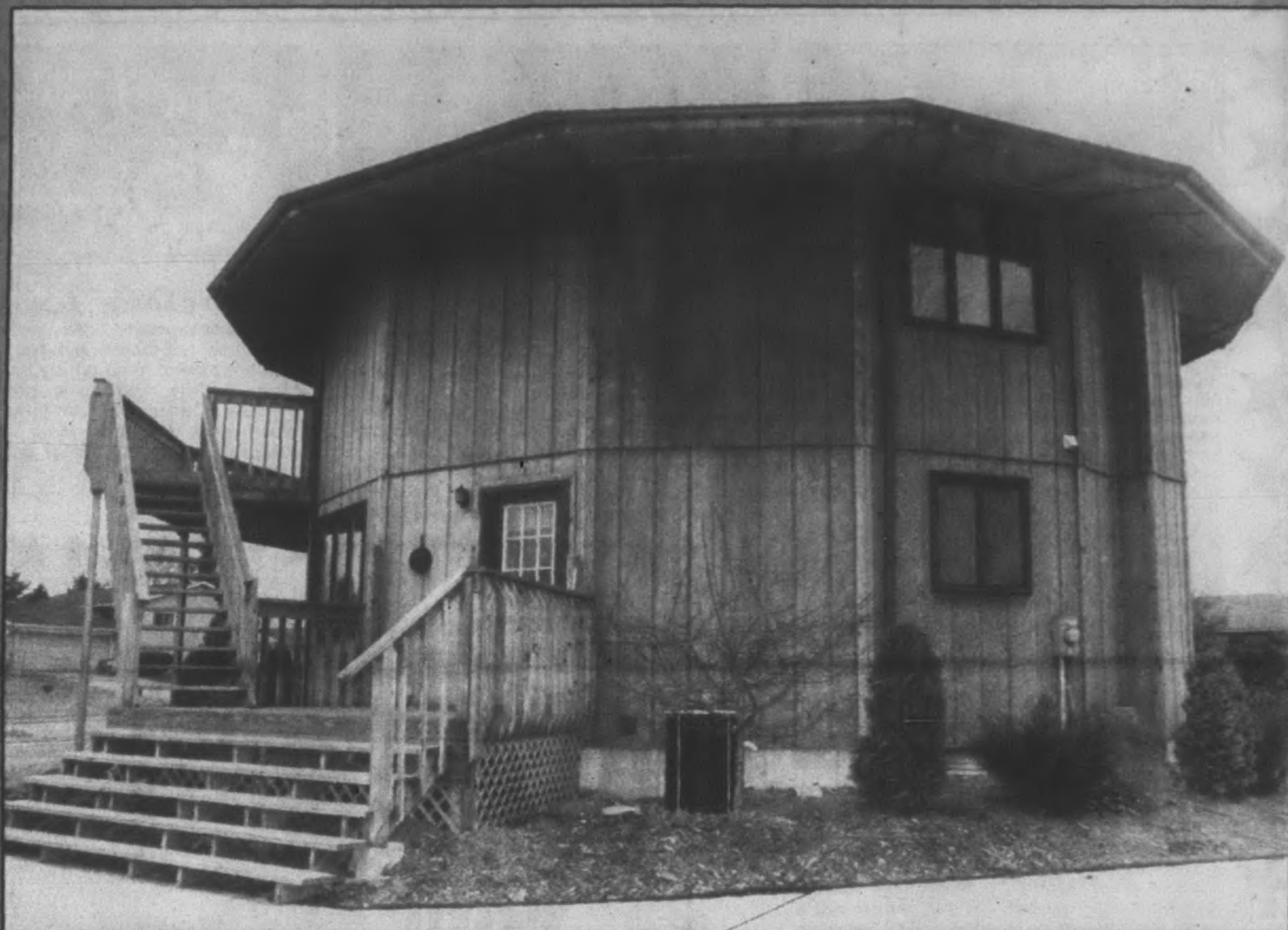
Bob and Corrine Dean's Eagle's Nest House includes 14 sides and a dome-style roof topped with a cupola. The Deans built the house of Douglas Fir with cedar-trim.
