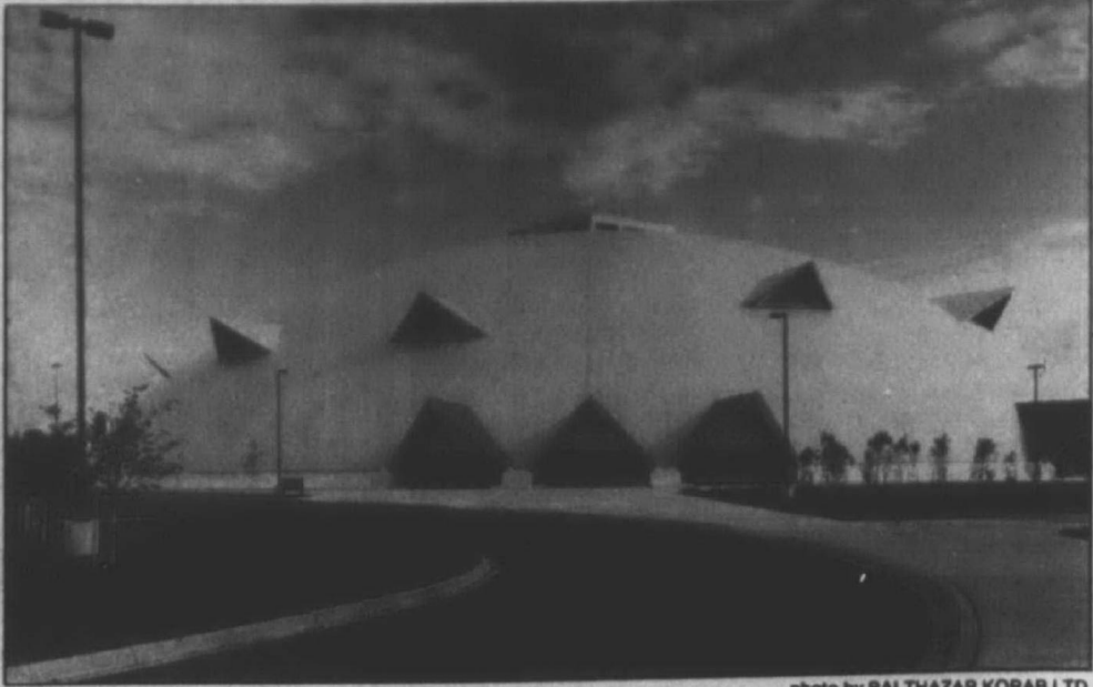
The Northern Michigan University Sports Training Complex was designed by TMP Associates of Bloomfield Hills. R.E. Dailey & Co. of Southfield was the supervising contractor.
