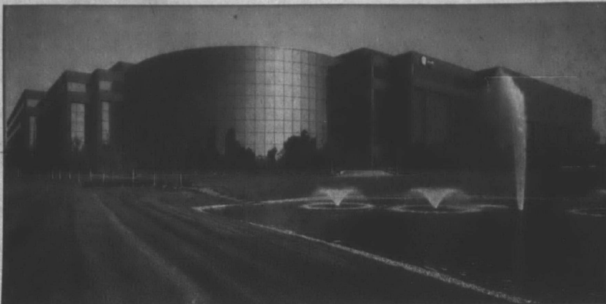
A.J. Etkin Construction Co. of Farmington Hills was the general contractor for the Volkswagen of America North American Headquarters in Auburn Hills.
