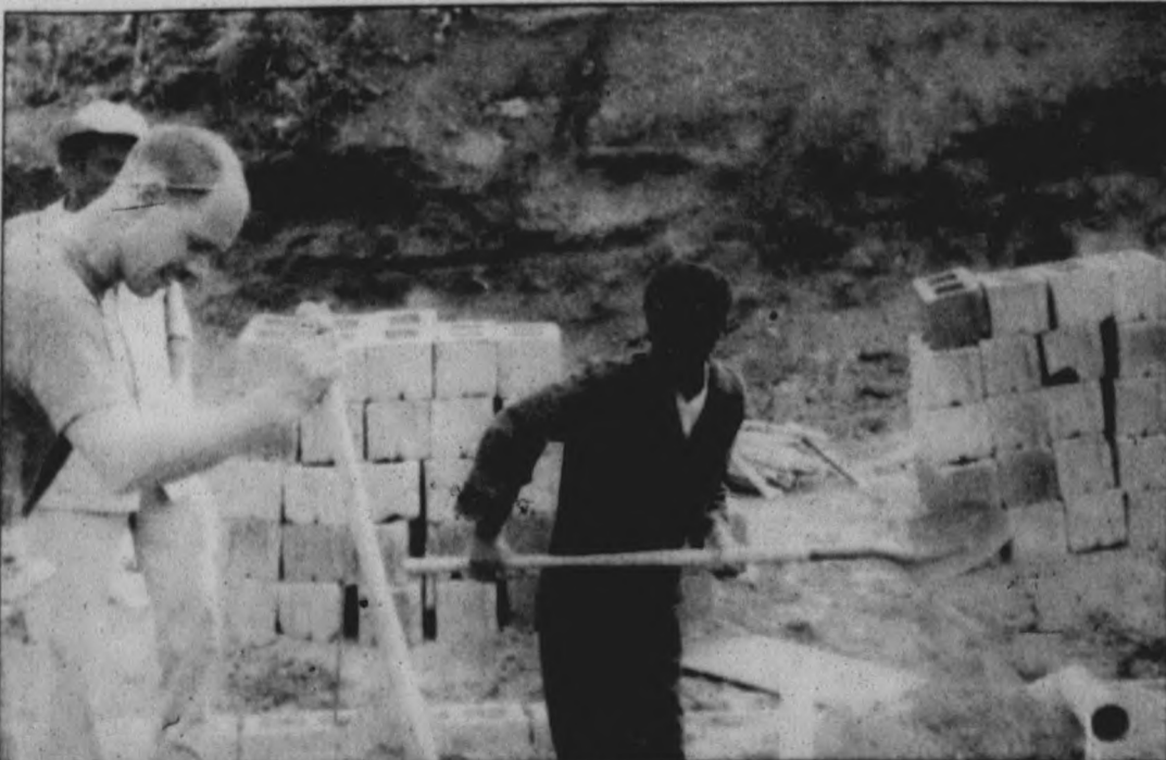
Plumber Scott Monroe of Wayne works with Ethiopian natives in installing drainage pipes under one of two buildings the team built in Kuriftu.
