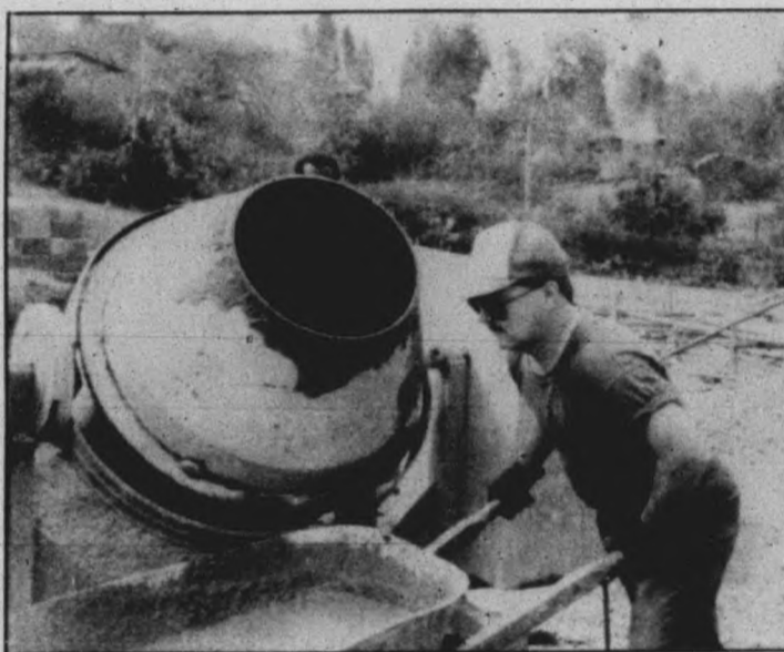
Bob Baker of Canton found himself on the heavy end of a wheelbarrow of cement during the construction work.
