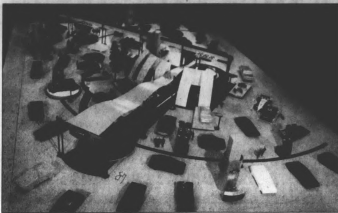
The 110' long x 24' wide x 20' tall exhibit, designed and produced by Livonia-based Exhibit Works, will be pulled from ground to standing at Cobo Arena in one fluid motion with the aid of two forklifts. This technology was pioneered by Exhibit Works in response to Ford's challenge to contain set-up costs. Traditionally, the upper reaches of an exhibit are assembled by workers hoisted on lifts.
