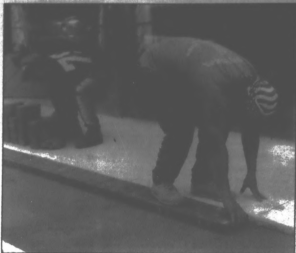
At work: Tony Dekinderen (left) and Shane Duffie lay brick sidewalk on Forest Street as part of the streetscape project. The old bricks have proven popular with local residents.
