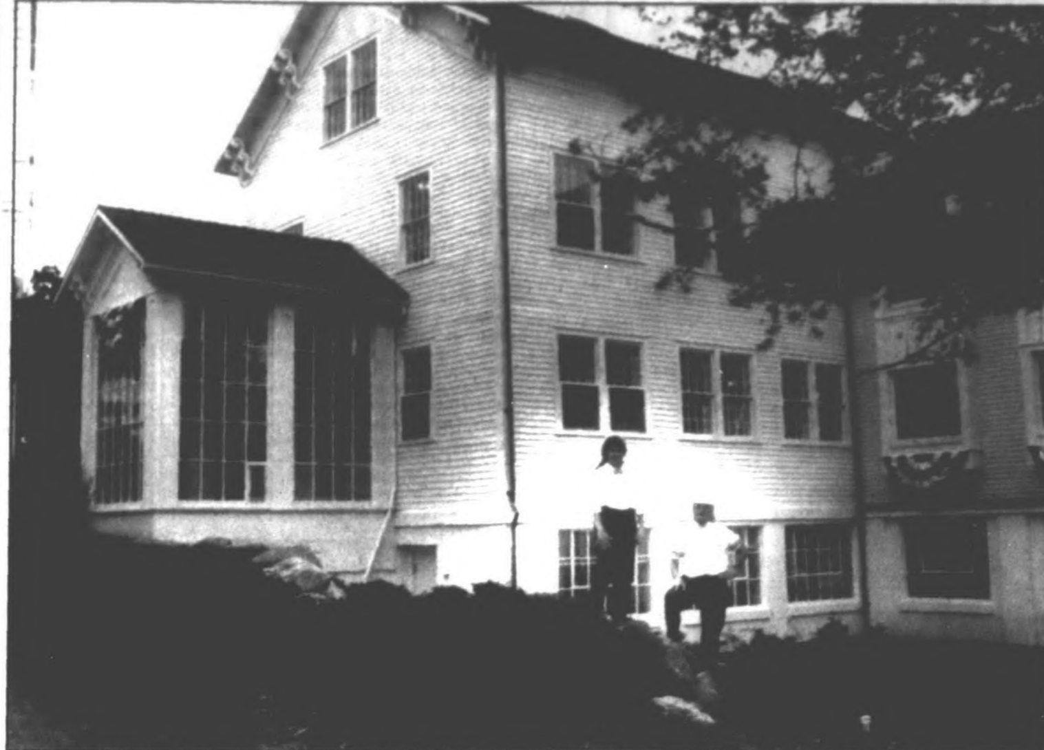
New office: Wayne County Parks staff members Tessie Pitses, manager of recreation and Skip Van Hooser, manager of parks, said they are looking forward to working out of the renovated parks office building and nature center on Hines Drive.
