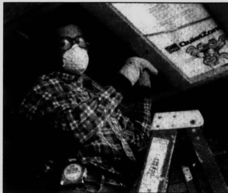
Making it quiet: Dean Johnson, host of public television's home-improvement show, Hometime , installs Owens Corning's QuietZone Acoustic Batts in a home theater construction. Installing acoustic batts in the frame cavities of interior walls and ceiling/overhead floors in one of the easier ways to control noise in a home theater.
