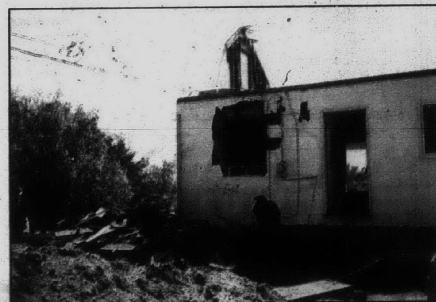
In progress: Walls were torn down and the house raised 16 inches to create a walk-out basement.
