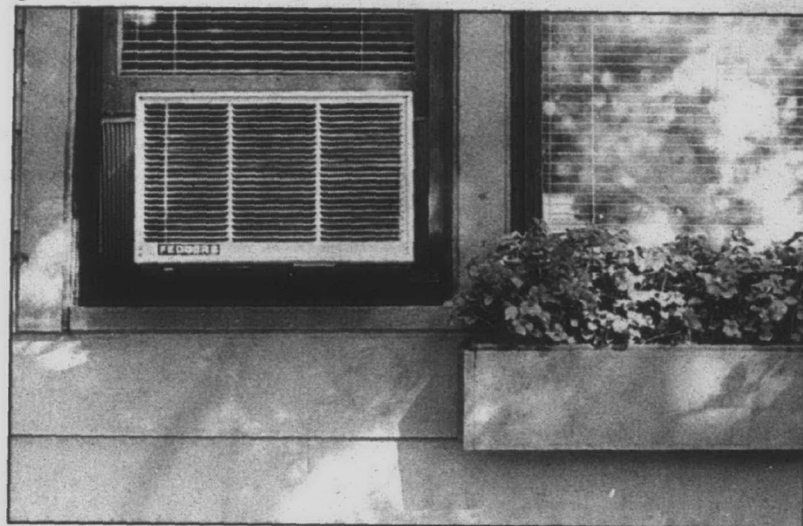
Directed cooling: Window units, less expensive than central air, can effectively bring down the temperature in a room or two.
