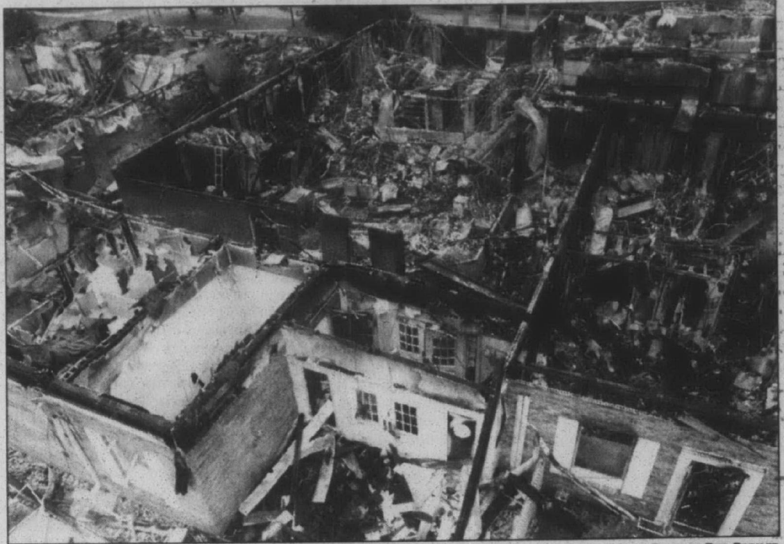
Aftermath: This is what's left of the 35th District Court building on Plymouth Road after fire, caused by an arc from wires that had fallen during the storm last week.
