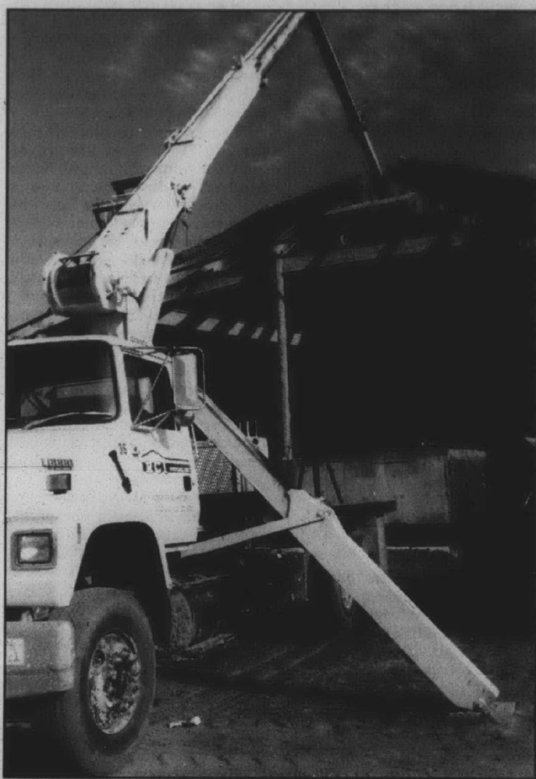
Accident: The boom (at right) on the construction crane bent in the middle and dropped the load. In the photo below, firefighters, EMS technicians, police officers and construction workers carry the injured worker to a waiting ambulance. The man was taken to the hospital and treated for a broken ankle.
