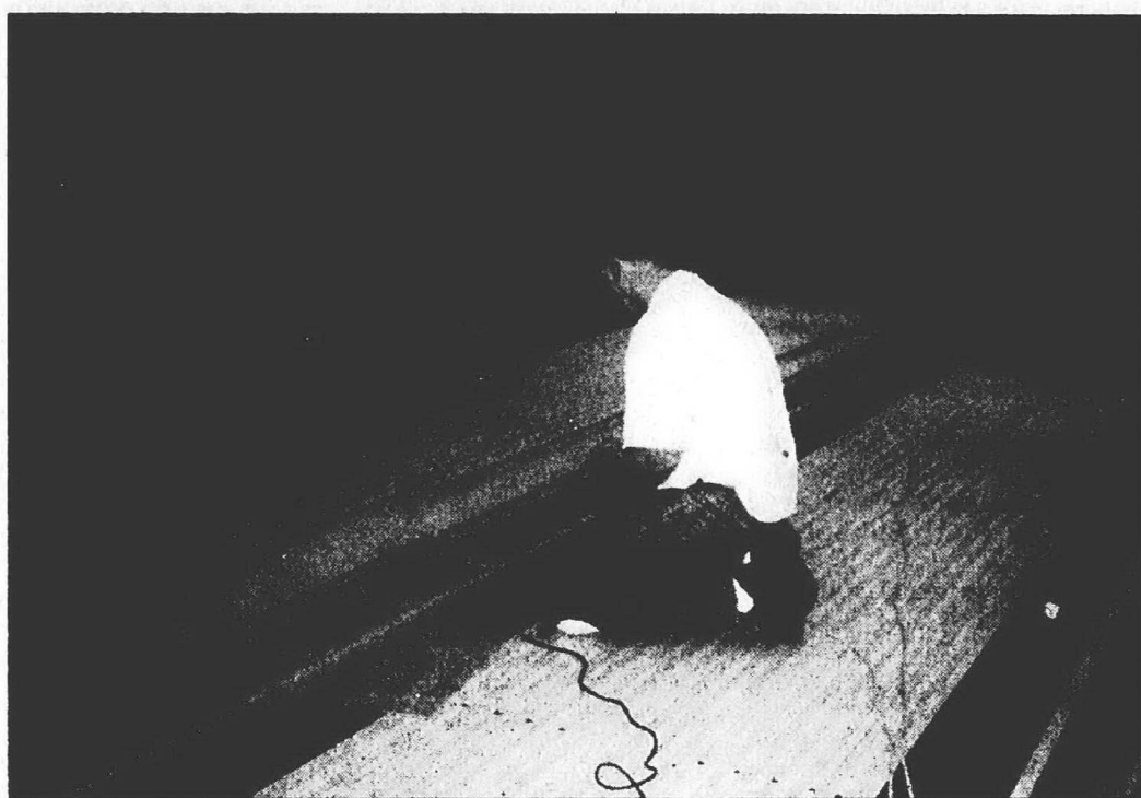
Precision counts: Installing Anvilanes, which Westland Bowl has just been outfitted with, is a precise and time-consuming job that includes making certain the sub-surface in perfectly flat.
