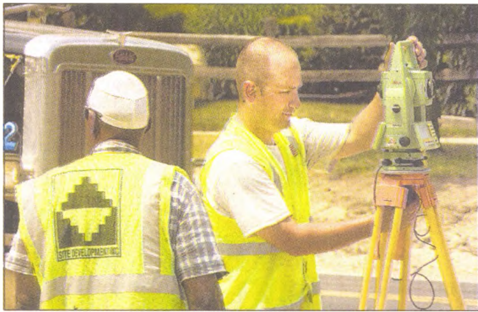
Leroy Wells and Michael McNutt, employees of the Wayne County Road Commission's field services, on the site of the Sheldon Center project.
