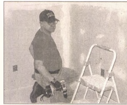
The Rev. Robert Brenner of Farmington First United Methodist Church works on a house in Mississippi.
