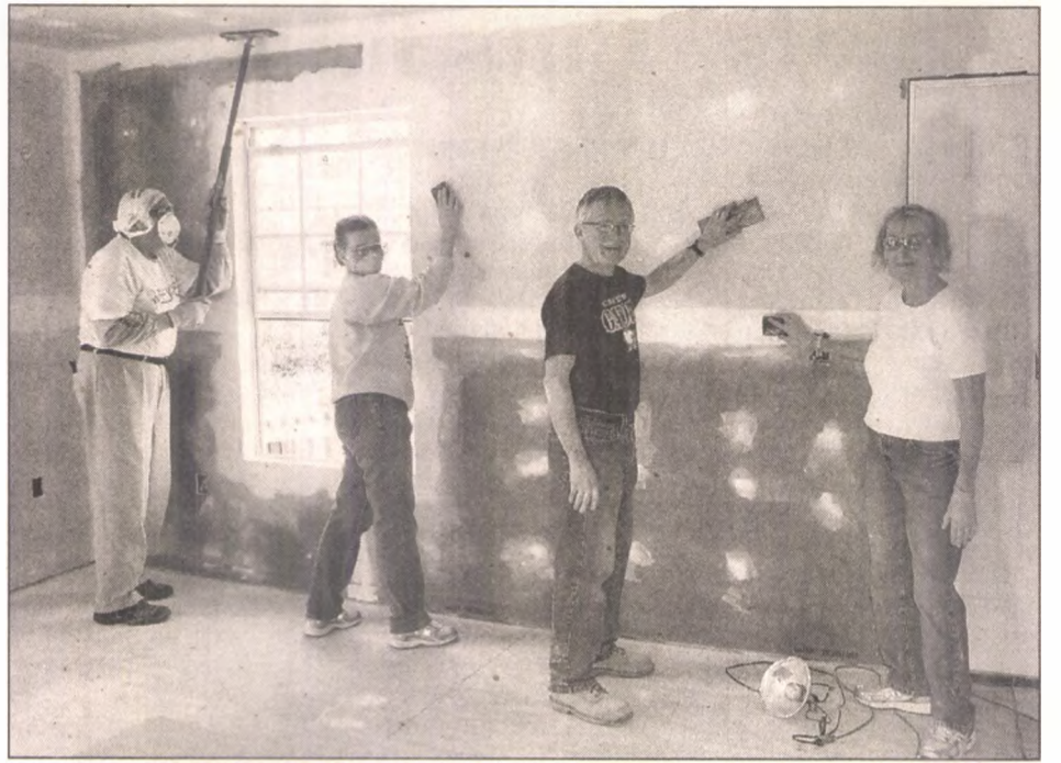
Volunteers from Farmington First United Methodist Church work on drywall in a home in Moss Point, Miss.
