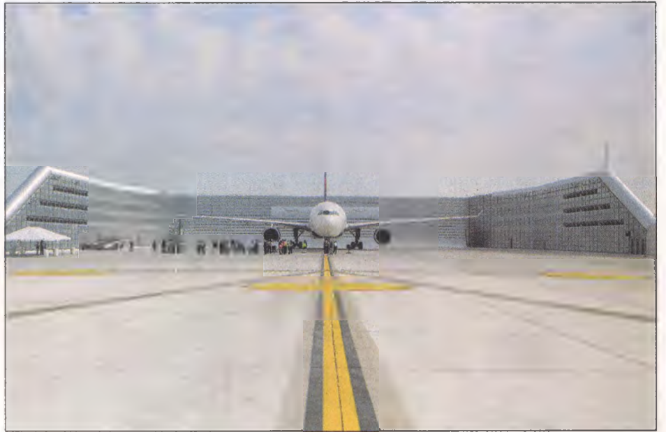
Airport and local officials are dwarfed by a Delta Air Lines A-330 in the new $11 million Ground Run-Up Enclosure dedicated Tuesday at Detroit Metropolitan Airport. The twin-aisle, wide-body aircraft, which is used on long-haul international flights, fits easily inside the GRE.
