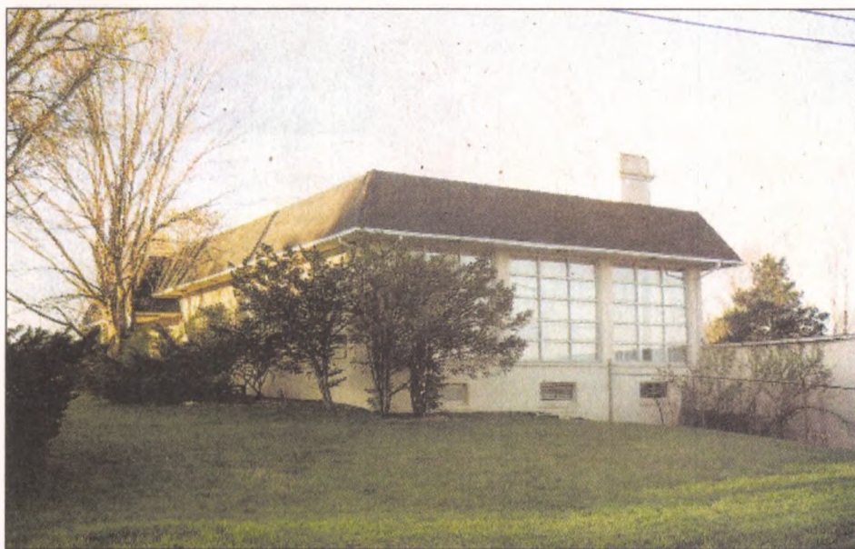
The Canton Partnership for the Arts and Humanities has begun building a business plan for the 50,000-square-foot Ford factory it bought last year.
