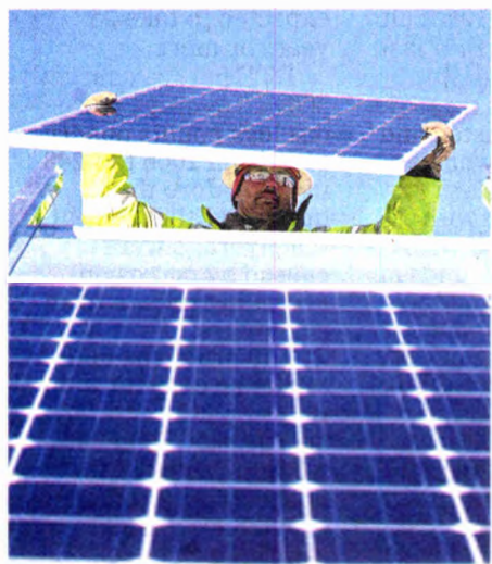
Electrician Bill Dillionson helps guide into place a solar panel at the DTE solar farm near Old Plank Road on March 3, 2014, in Lyon Township.
