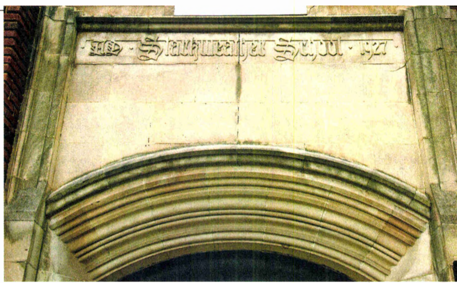
The former Starkweather School has two entrances.
