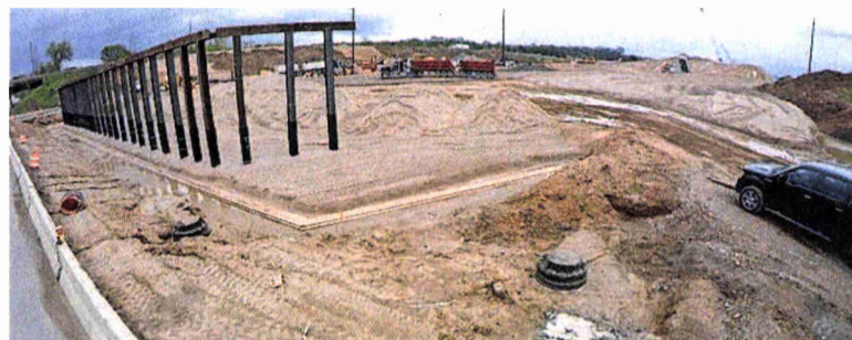
GILLIS BENEDICT | MICHIGAN.COM Construction of the Interstate 96 and U.S. 23 interchange continues.
