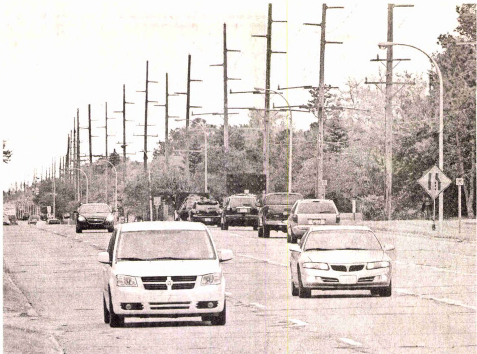
Cherry Hill Road will be rebuilt from Merriman to Wayne Road running through Garden City and Westland.
