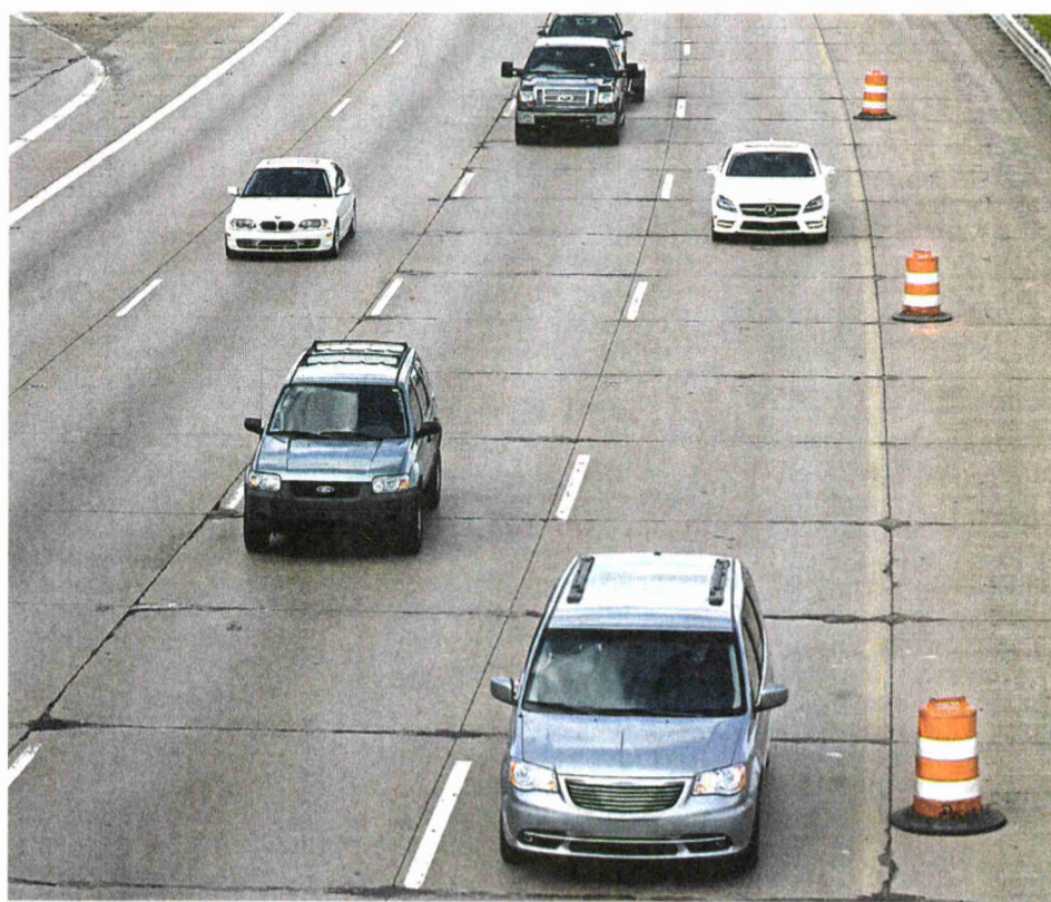
JOHN HEIDER | STAFF PHOTOGRAPHER Orange construction barrels line the side of the road of southbound I-275.
